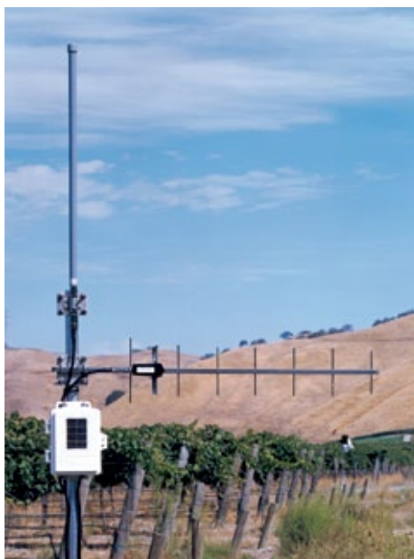
Long-range repeater with one Yagi and one Omni antenna.
